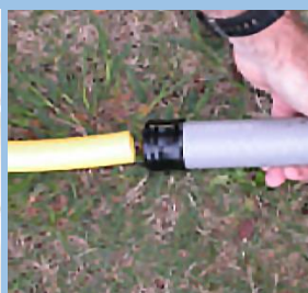
3. Insert the plastic tubing through the moisture seal at the opposite end of the riser casing. Allow the tubing to extend at least 4" past the nut.
