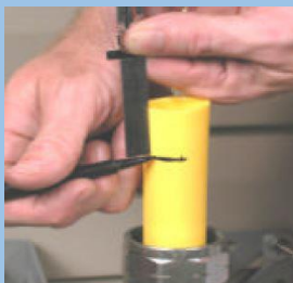
6. Measure and mark the correct stab depth length on the plastic tubing (see stab depth chart above). Make sure not to scratch or damage the surface of the tubing.
