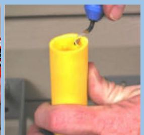
5. Remove burrs from pipe O.D. and I.D. Clean pipe thoroughly to ensure there is no dirt, grease, oil, or other contaminants on the assembly area.
