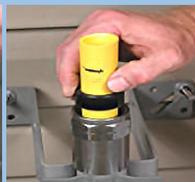
7. Ensure the gasket is free of debris and slide it over the plastic tubing and into the nut. Make sure the gasket is securely seated in the nut.
