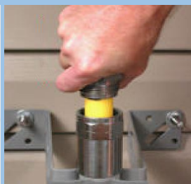
9. With the body/stiffener assembly positioned in the plastic tubing, force the tubing down into the riser casing until the SHA body and nut are in contact.
