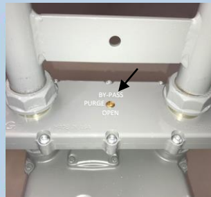
2 Turn the Co-Pilot to BY-PASS
