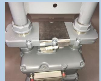
8 Lock the security cover plate
